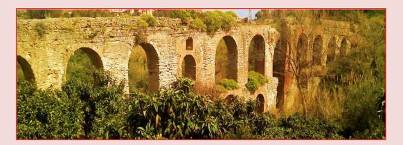
**Romanic Aqueduct** Built in the second century A.D., rappresents the largest and unique in its kind Roman architecture in Sicily. The massive hydraulic work consisted of a long and complex aqueduct system that from the source reached the top of the city. It works up for over 100 feet in length and for a maximum height of 16 meters. The bridge is constituted by a double series of arches. *Contrada Figurella*.
